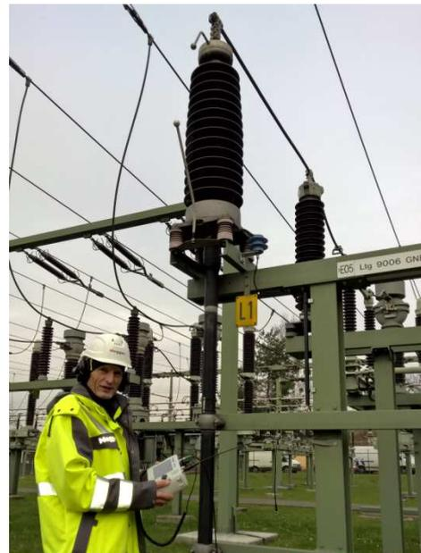
**Figure 12 onsite UHF measurement**
